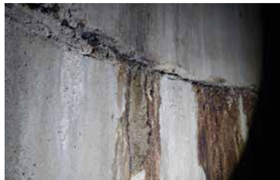
Figure 19 – Cracks in the lining of shaft 1 through which limited amounts of water enter the shaft
