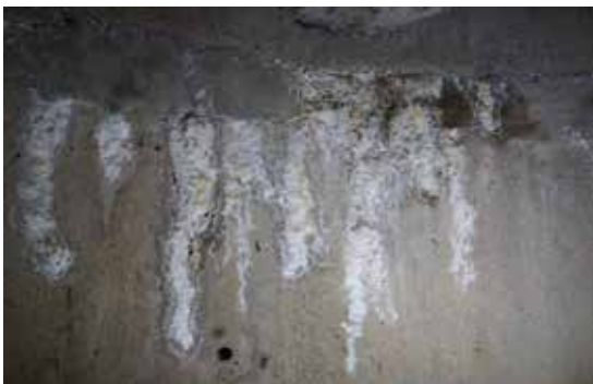
Figure 19 – Cracks in the lining of shaft 1 through which limited amounts of water enter the shaft
