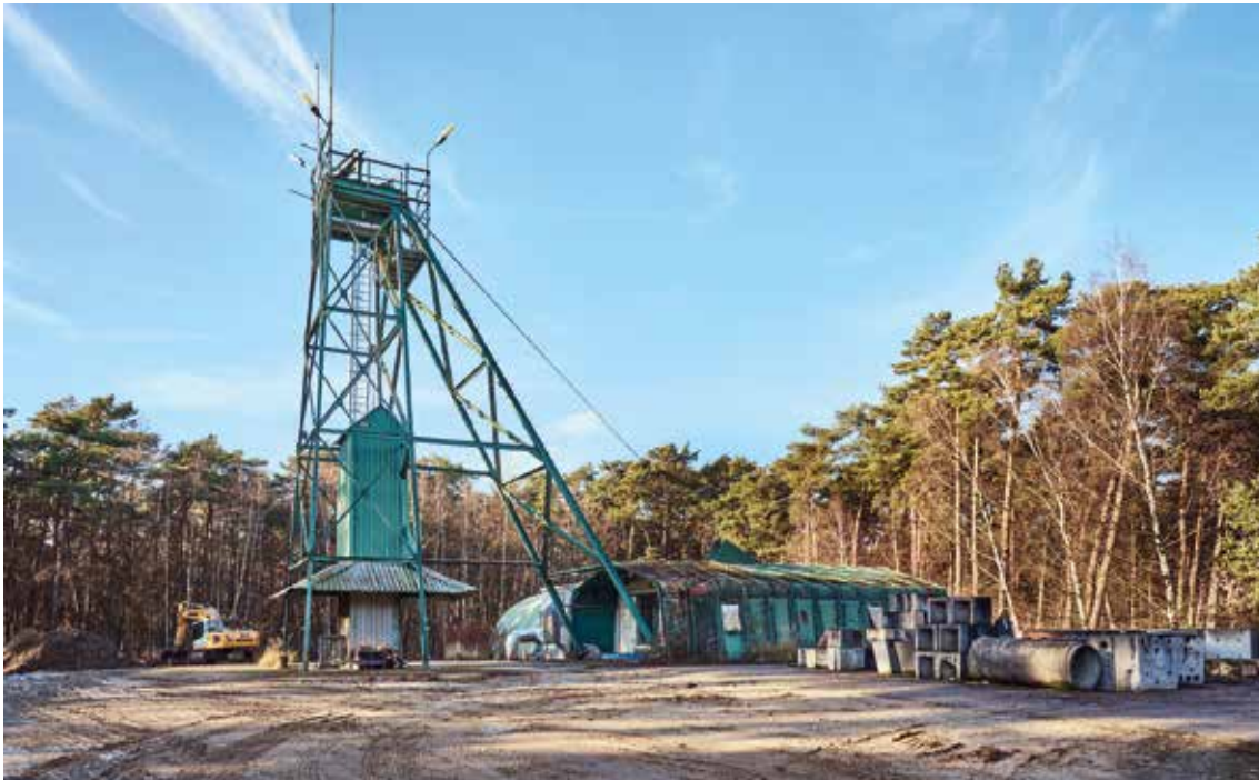
Figure 18 – Hoisting tower and machine room of the old hoisting system of shaft 1
