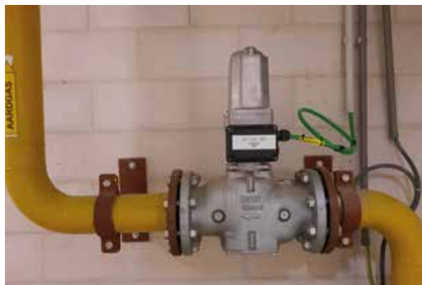
Figure 17 – Automatic gas valve connected to the existing gas detection and fire control panel
