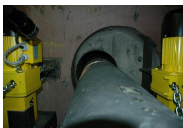
Figure 24 Installation of FORGE packer system
